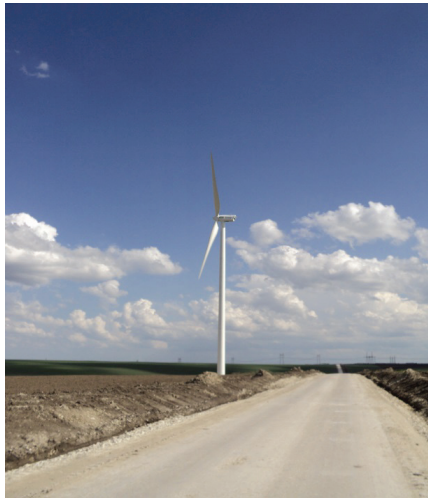
Figure 18. The road Pestera Wind Farm after the execution
