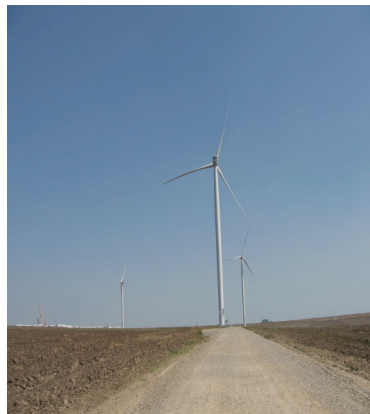
Figure 16. The road of Wind Farm Fantanele after the execution
