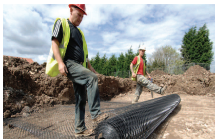
Figure 13. Easy to install triaxialgeogrid.
