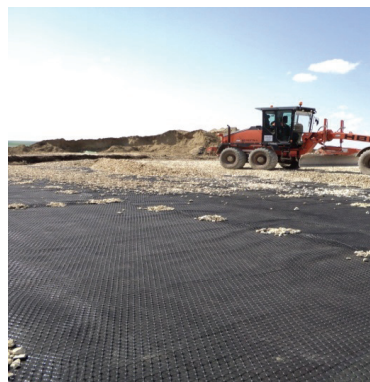
Figure 17. Relevant photos during the execution Pestera Wind Farm
