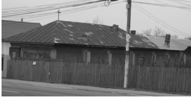
Figure 2. Strengthening of the external walls with some buttress to a traditional dwelling
