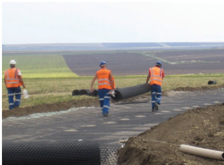
Figure 15. Relevant photos during the execution Wind Farm Fantanele
