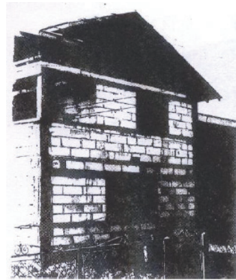
Figure 4. City type rural two storied yong blocks dwelling with RC members (RC window beam lintel parallel to the collar beam and floor slab acting as a frame with columns; foundation is made of concrete)
