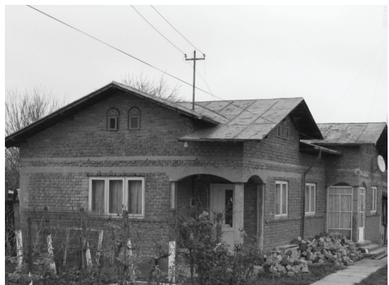
Figure 6. City type rural two storied brick masonry dwelling with embedded RC columns and RC slabs (the collar beam as a frame beam)
