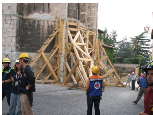
Figure 4. Emergency measures to secure a building after earthquake
