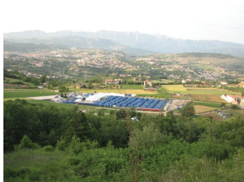
Figure 3. Camp tent near L'Aquila town
