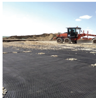
Figure 17. Relevant photos during the execution Pestera Wind Farm
