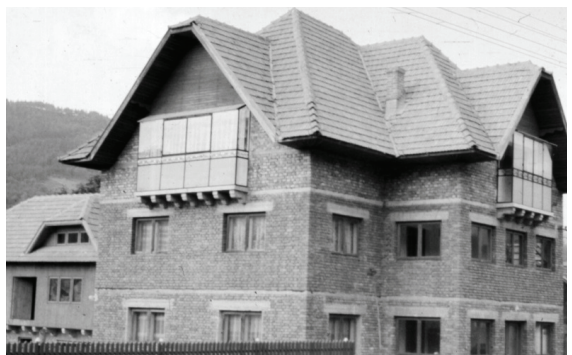
Figure 12. City type rural three storied brick masonry dwelling with RC floor slabs and without RC belts
