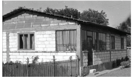
Figure 10. A traditional dwelling with RC floor slabs (lintels are embedded in RC floor slab)
