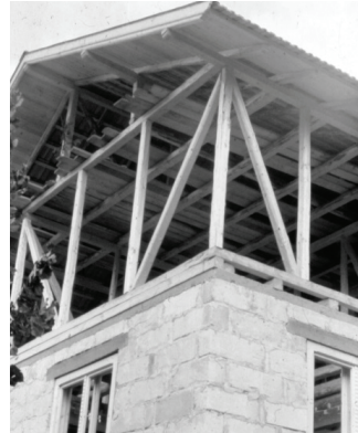
Figure 8. A traditional dwelling with roof band and RC lintels, without pillars at corners, a light roof, in 2-4 slopes having a structure well tight with the masonry
