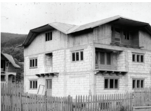
Figure 11. City type rural three storied brick masonry dwelling RC skeleton mixed with timber beams
