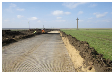
Figure 20. Relevant photos during the execution road Chirnogeni Wind Farm
