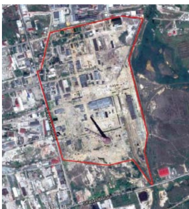
Figure 3. Satellite view of Cuprom area ( https://www.google.ro/maps/@47.6545769,23.601314,1415m/data=!3m1!1e3?hl=en )
