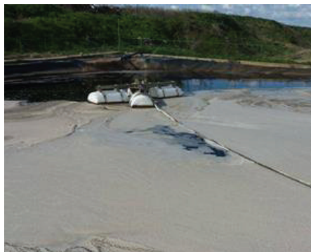
Figure 2. Aeration lagoon of the landfill Glina
