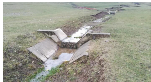
Figure 3. Land reclamation works in Inucu area
