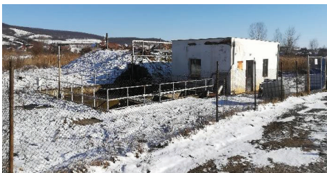
Figure 1. Sewage treatment plant from Aghiresu-Fabrici
