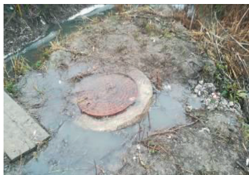
Figure 3. The discharging of the untreated water from a waterway mouth located by the Daia creek
