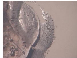
Figure 6. a. A tsunami floods over the breakwater protecting the coastal city of Miyako – Japan 2011 [9]; b. Earthquake-related failure of the breakwater in the Navlakhi port in 2001[10]
