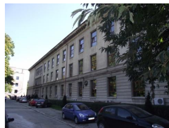
Figure 2. Main facade of Horticulture Faculty building
