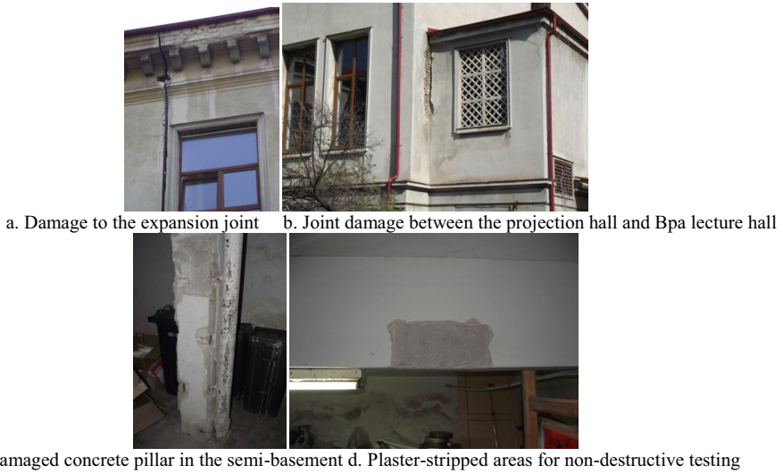
Figure 4. Main structural damages of the Horticulture Faculty building
