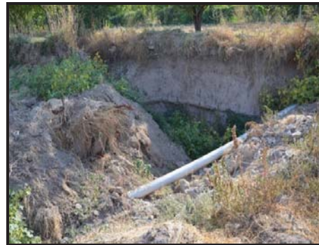
Figure 11. İçeriçumra Abaz Sinkhole plugged following its emergence
