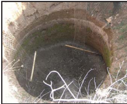
Figure 10. İçeriçumra Çakillar Sinkhole-I plugged in present day (Photo taken in 2008)
