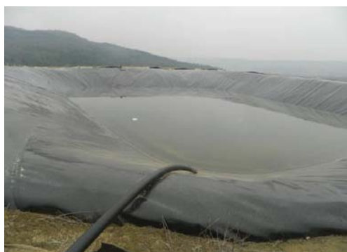
Figure 5. Storage and water heating tank
