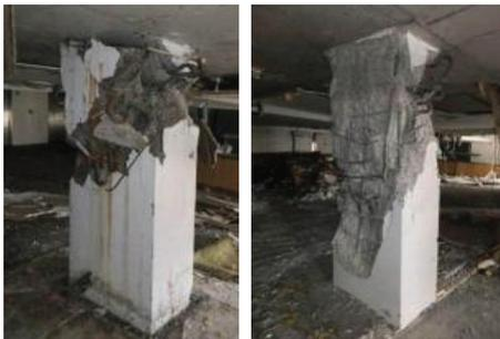
Figure 25. Grand Chancellor Hotel: The shear-axial failure of the RC columns below the transfer girders at Level 10 and 11.
