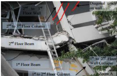
Figure 16 a. Various failure mechanisms observed on the Northern elevation of the collapsed PGC building (<http://www.nzsee.org.nz>)
