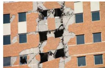
Figure 9. Details of facade failure, high axial/shear and bending forces (Decanini, 2010)
