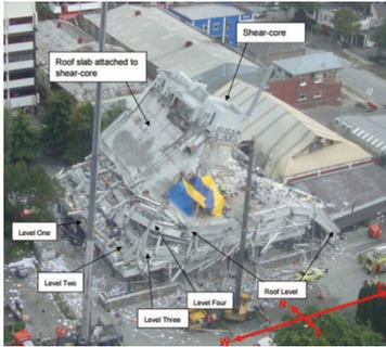
Figure 14. General Location of Main Structural Components after Collapse (<http://www.building.govt.nz>)
