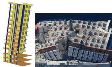
Figure 4. Damage modelling and view of collapsed building (<http://www.nehrp.gov/pdf>)
