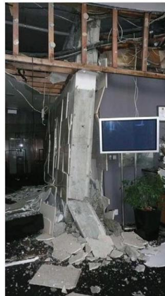
Figure 22. Shear wall D5-6 base failure. A lack of steel reinforcing in the concrete was the biggest factor in the shear wall's failure which failed in a brittle manner. This shear wall had supported vertically approximately one eighth of building's mass and was also expected to carry a portion of lateral earthquake loads
