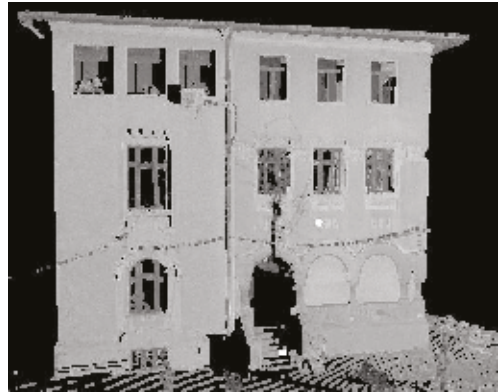
Figure 8. Point cloud of the facade
