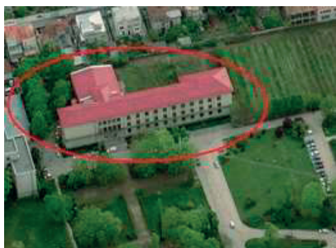
Figure 2. The building with the two sections, B1 and B2
