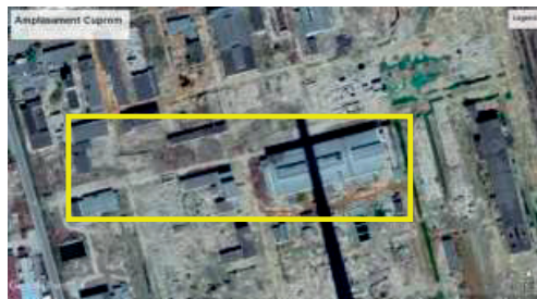
Figure 1. Research area (image source: Google Earth)
