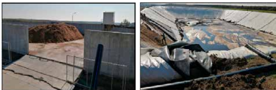
Figure 3. Solid dejections storage platform and waterproof lagoon for liquid dejections storage
