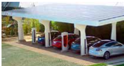
Figure 6. Power supply stations ( https://cleantechnica.com/2012/08/26/solar-powered-electric-vehicle-charger-launched/ )
