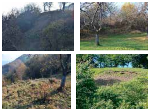
Figure 3. Landslides identified on the Location 6. Cămpul Negru - Malec
