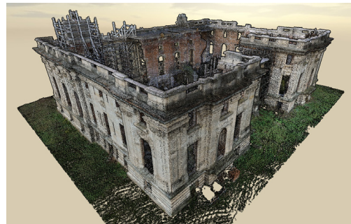
Figure 9. The complete digital model of the Little Trianon Palace - Potree-Prosig visualization
