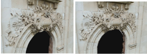
Figure 13. Modelling the bas-relief on the southern facade: based on images (left) and based on LIDAR and Images (right) - 3DF Zephyr
