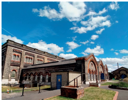
Figure 1. Crossness Pumping Station (© 2023 Elena Nistor All Rights Reserved)
