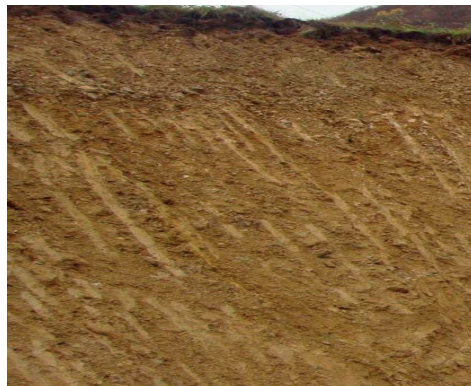
Figure 5. Soil profile on rupture terrain with accelerated erosion
