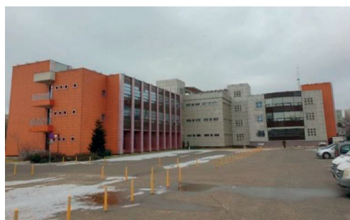
Figure 5. The building of the Faculty of Biotechnologies. Year of construction 2016, S+P+2E, reinforced concrete structural frames and walls, Granite instrument type
