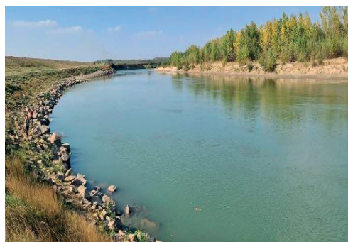
Figure 8. Anti-erosion works carried out in the area
