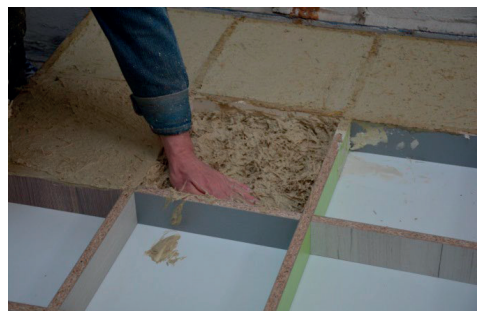
Figure 2. Filling the formwork with mixture
