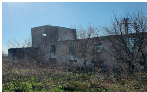
Figure 2. Overview of the SPP15 pumping station OUA1 Hotarani Mehedinti County
