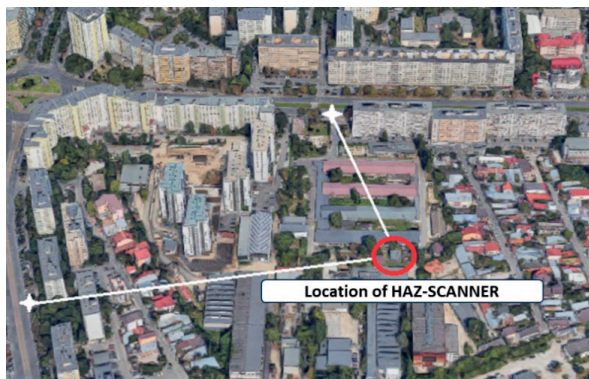
Figure 2. HAZ-SCANNER equipment position compared to the two boulevards
