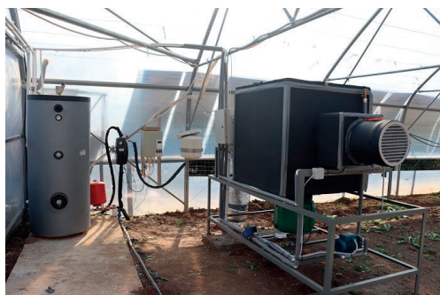
the indoor unit and the puffer
