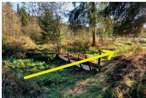
Figure 3. The barrage built to limit the water flow from the BBN peatland (arrow - the flow direction of the drainage ditch towards DC 85B and the Bancu River)
