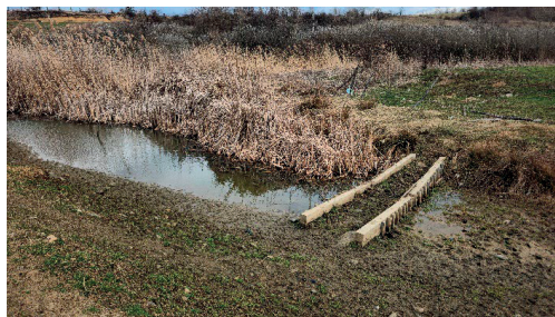
Figure 10. Blockage of the drain channel (13.03.2025)
