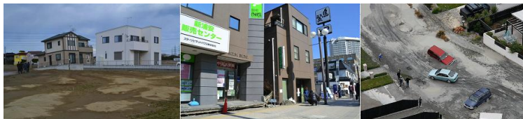
Figure 4. Damage due to soil liquefaction and permanent settlement [8]
