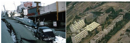
Figure 5. It is showed how buildings can topple when soil assumes the properties of a liquid and loses its bearing capacity [8]
